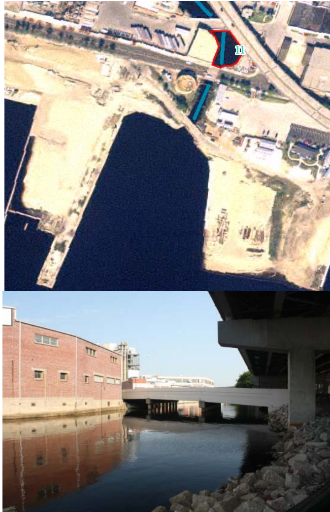
Figure 15: Restoration area 11 is located north of Bay Street and west of Hart Expressway.
